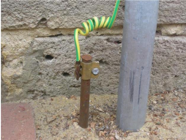
The neutral/ground connection also connects to one or more earth ground rods driven into the ground near the service meter similar to the Australian example grounding rod shown at left. The ground circuit may additionally connect to the cold water pipes that service the building. This is how each branch circuit gets its connection to earth ground (the AC neutral coming from the utility pole is also earth grounded near the pole).
